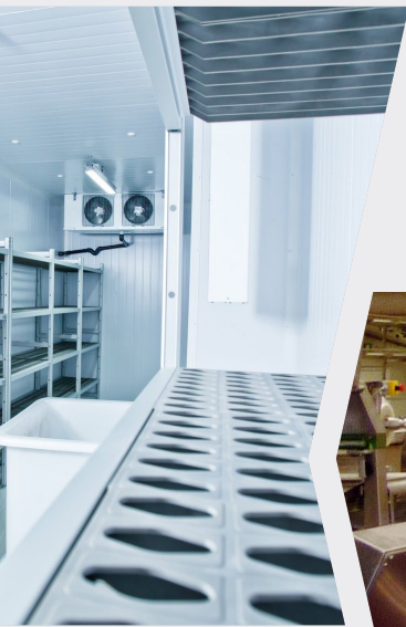
Cold storage cells (0 °C / +8 °C) Blast chilling cells
